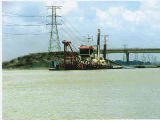
IHC Beaver 50 Cutter Suction Dredger at work.
